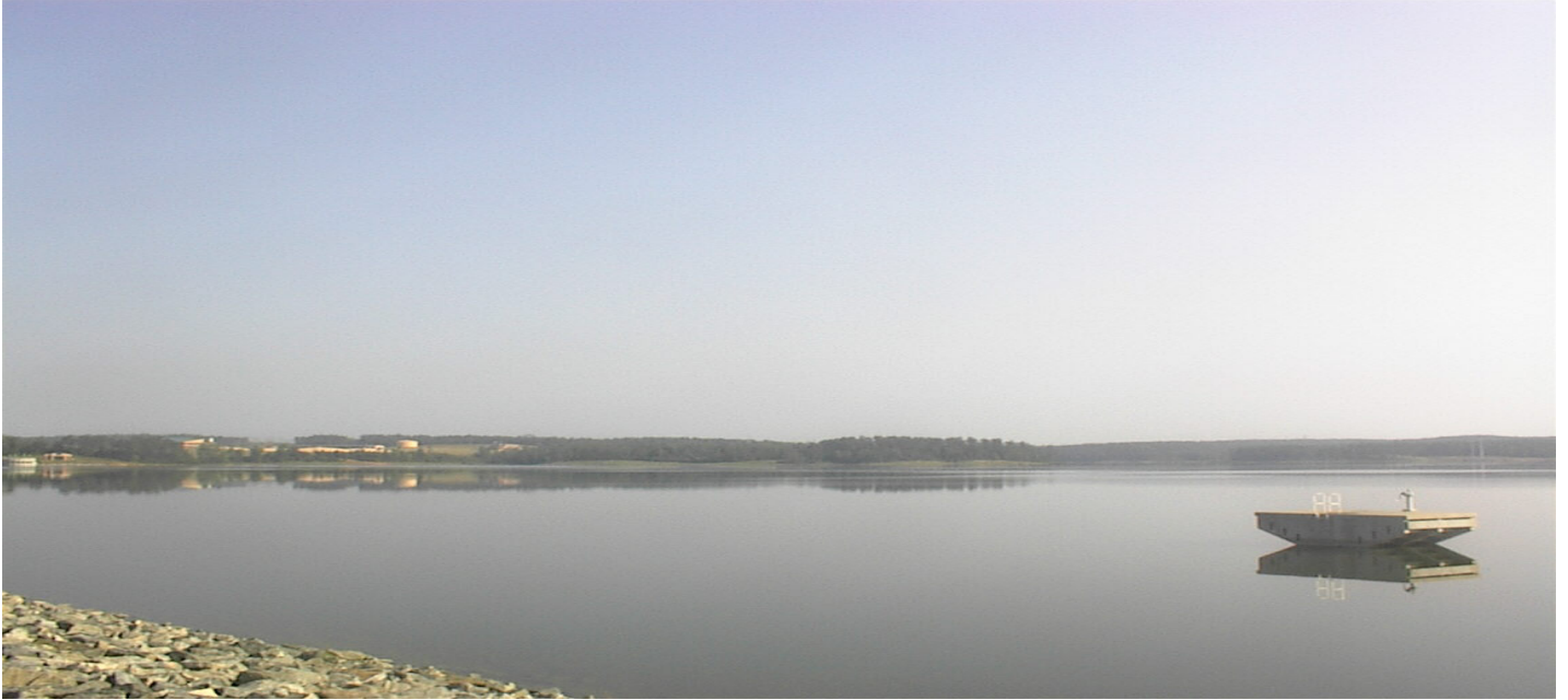
View of Town Creek Reservoir from Dam
