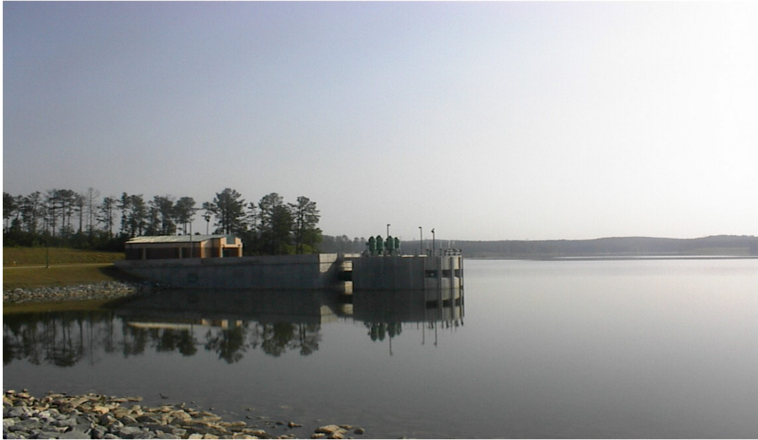
Town Creek Reservoir Pump Station
