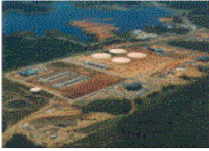
The new Town Creek Water Treatment Plant, scheduled to come on line in February 2000.
